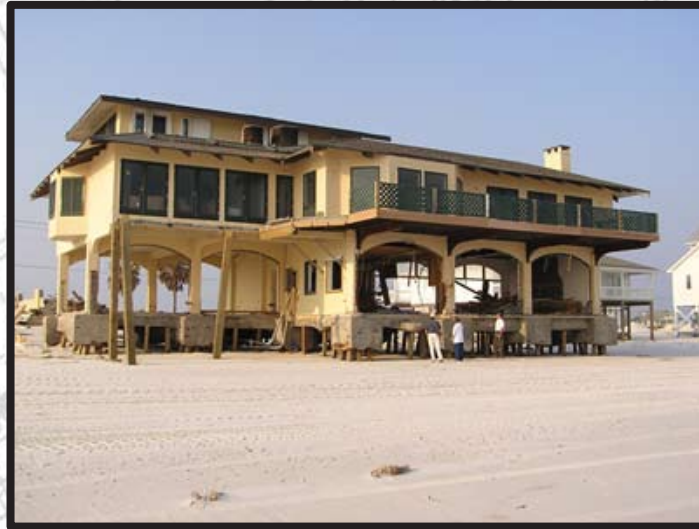
Company Engineers Inspect Residence in Gulf Shores
